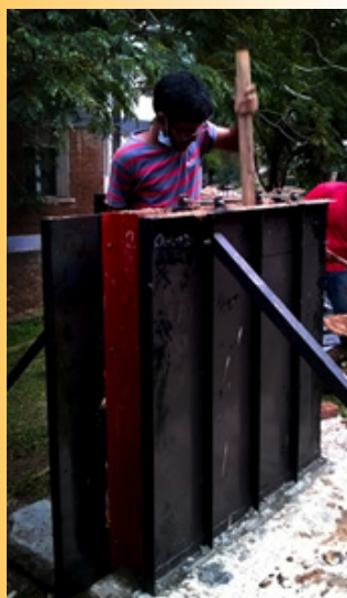
Assembling the frame work-Process of in-situ cast mud-concrete wall construction
