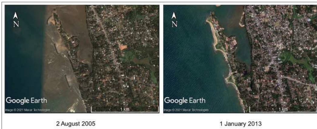
Figure 10: Satellite images of a detached breakwater on 2 August 2005 and 1 January 2013 in cell 5 (Source: Google Earth Pro, Maxer Technologies)
