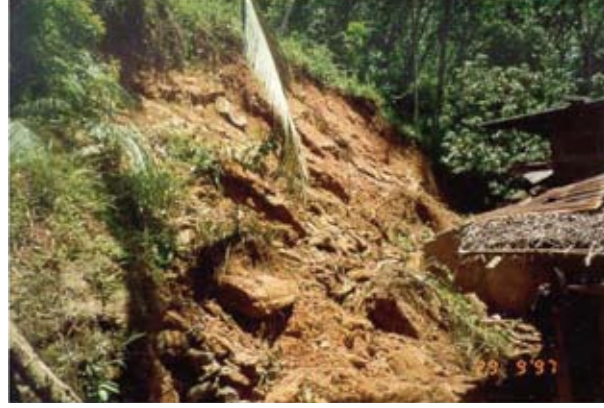
A damaged house due to a landslide at Yatiyantota
