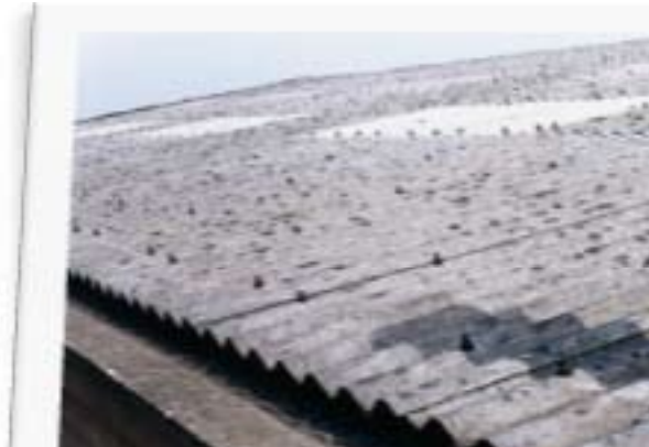
Asbestos is a popular roofing material
