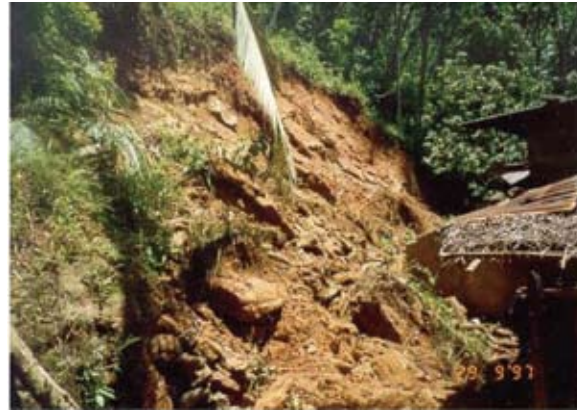
A damaged house due to a landslide at Yatiyantota
