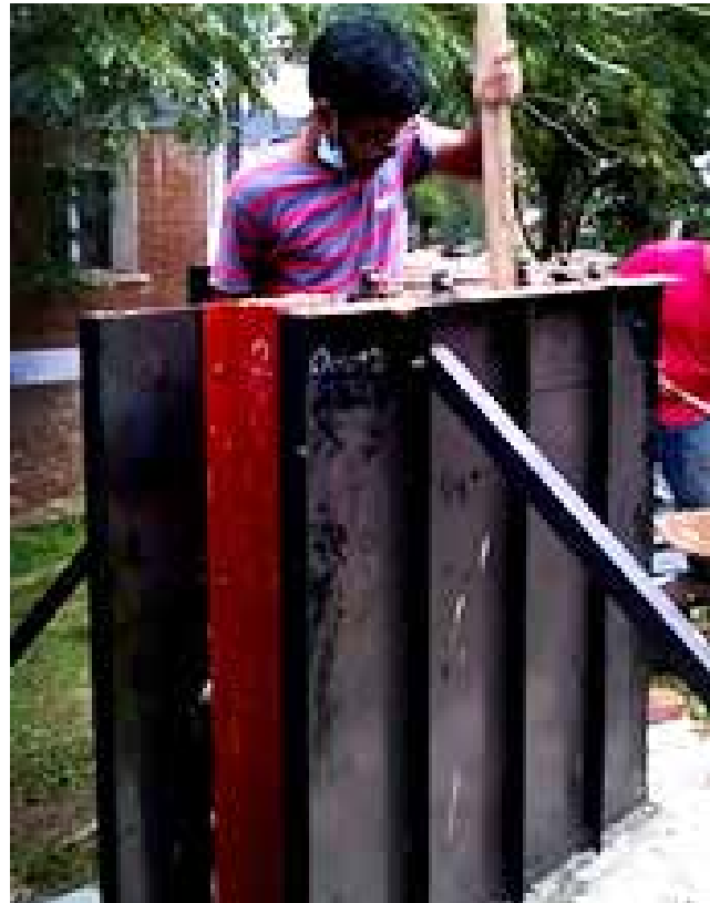
Assembling the formwork - Process of in-situ cast Mud-Concrete wall construction
